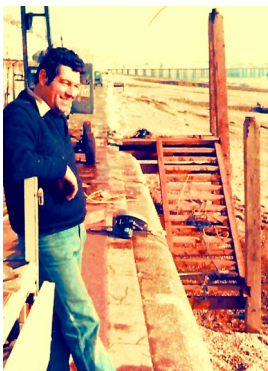
Brian at work on Hastings promenade, installing a new set of steps
